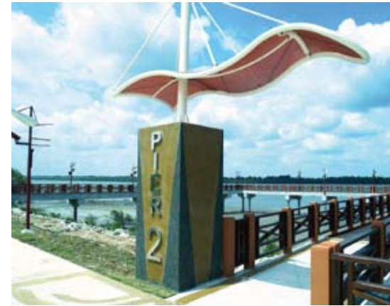
Pier 2, Laguna Park
