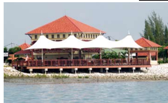
Pier 1, Laguna Park
