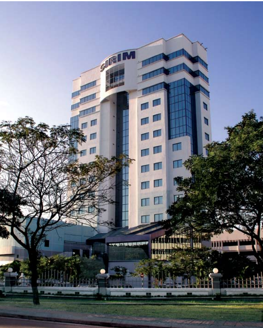
Sirim Headquarters at Shah Alam
