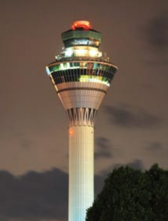
Operating tower at KLIA
