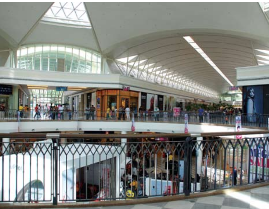
An intricate roofing detail.
